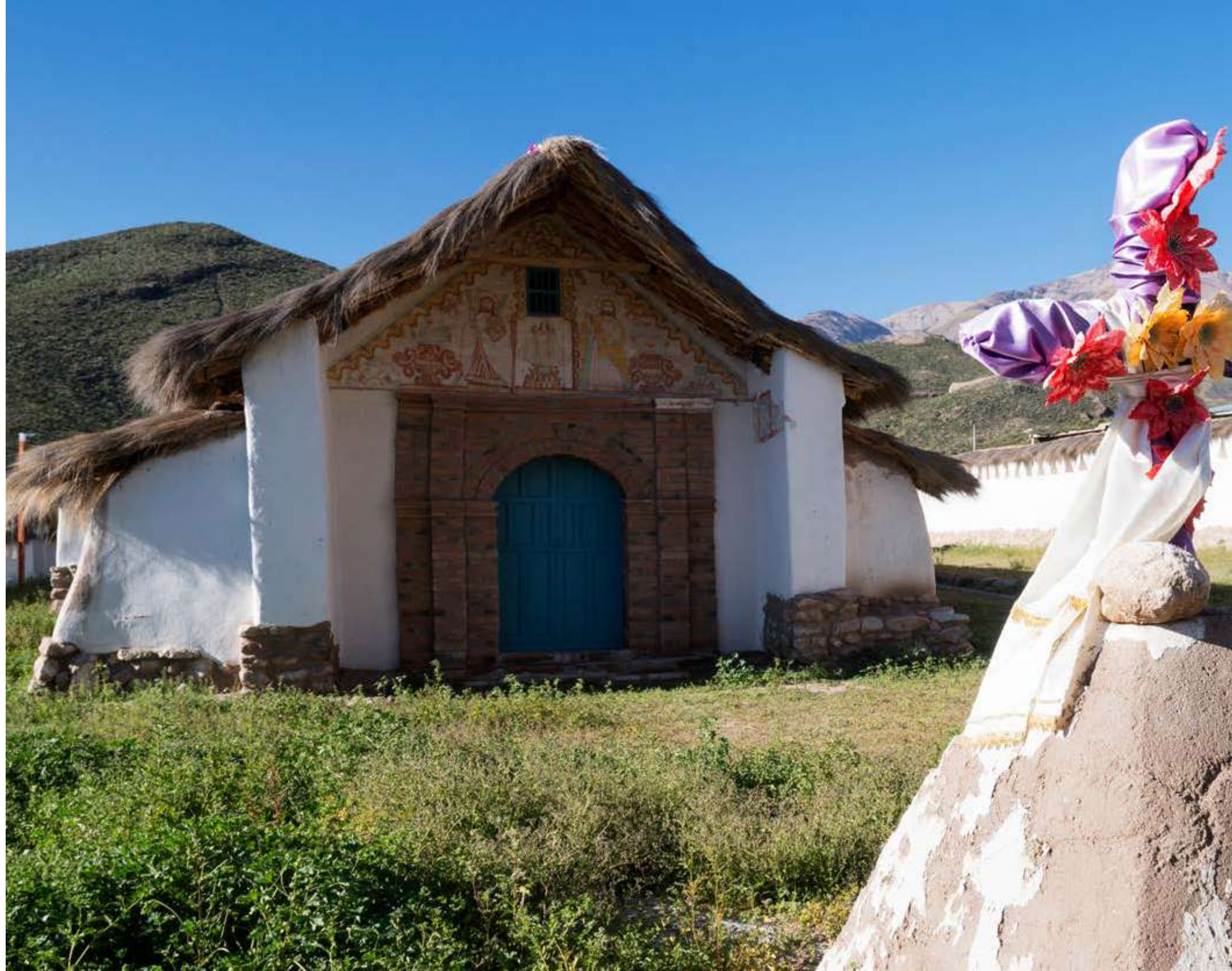
Vista desde el atrio, templo de Pachama restaurado. View from the atrium, Church of Pachama, restored.
